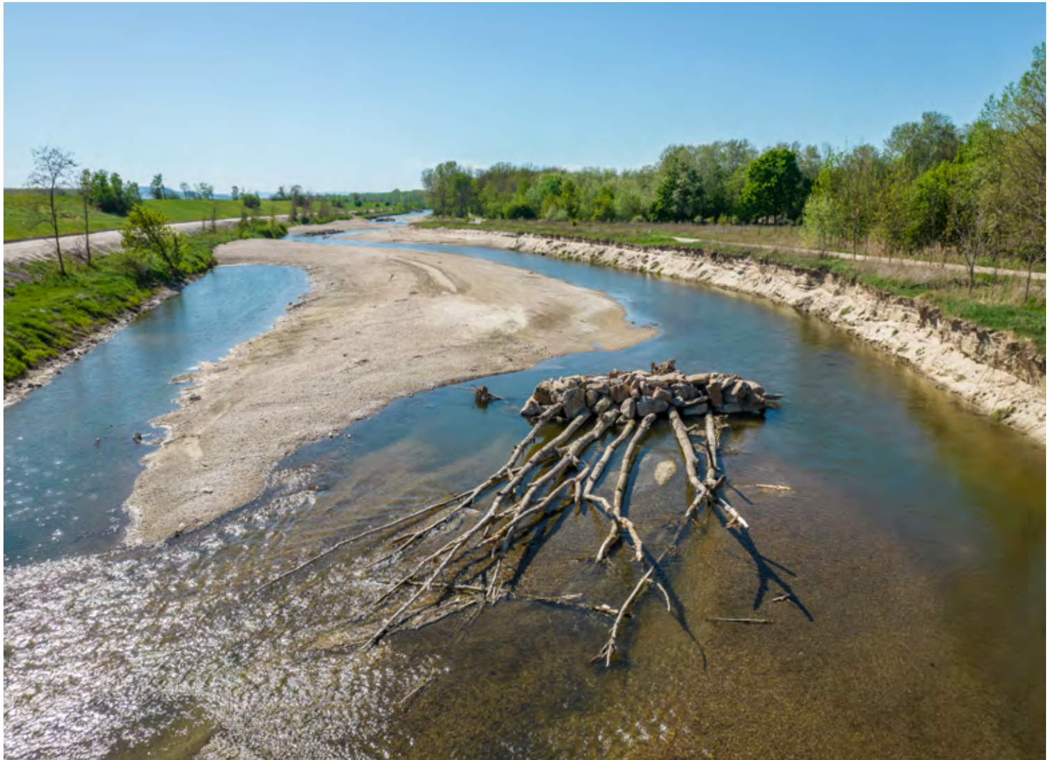
Altenwörth dynamic bypass river: about 30 hectares of new river habitat have been created in the LIFE Network Danube Plus project.
